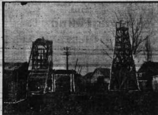
The Bean street shaft, on the northwest sewer. The above picture shows the shaft from which gangs will work north to the tunnel already partially pierced under Sunnyside from the Victoria Arm, and also drift south towards the open cut on Hereward road. The latter will pass under houses at Belton avenue and Pine street, connecting at Hereward road with the drift from the shaft at the intersection of that road with Wilson street.
